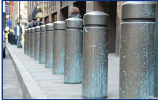
K-rated bollards create a hard perimeter.
